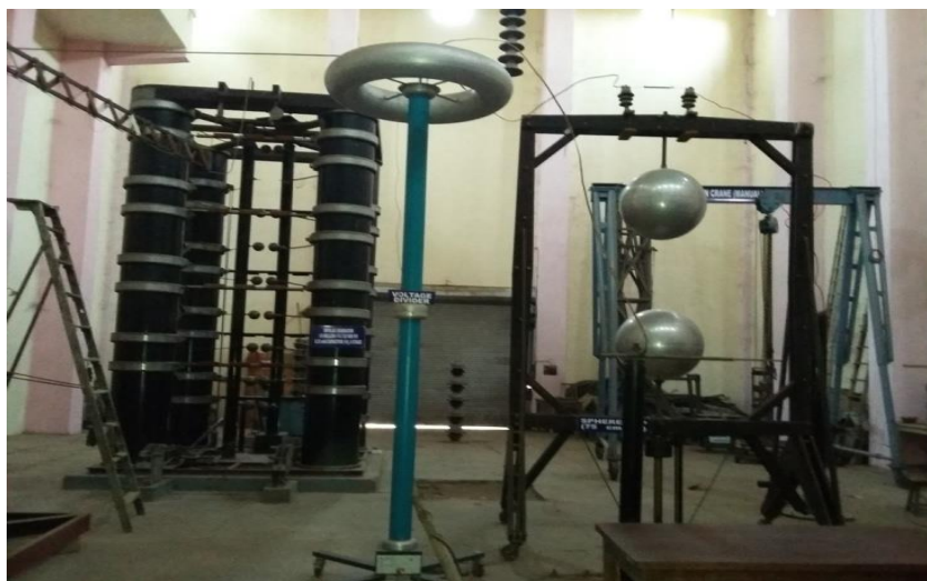
SETUP OF IMPULSE GENERATOR
